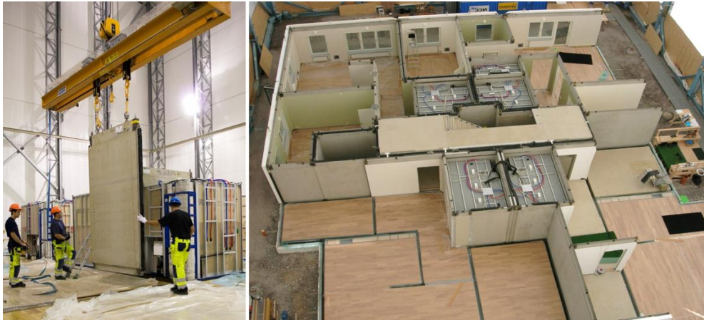
Figure 7:11 Final assembly process within the mobile assembly hall to left, and the half-way finished floor to the right. Note that the assemblers are working white gloves “on-site”.
